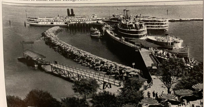
EXCURSION BOATS AT THE DOCK — PLAYLAND, Westchester Co. Park System, RYE, N. Y. Another way to come to the park was via boat. Before small ferries came to the shorefront of Rye landing at Dearborn Avenue, but now people came by much larger boats, almost liners in service to Playland from New York City and Jersey City. Round trip was $1.75 for adults and 70¢ for children.
